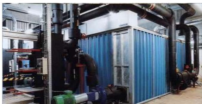
Figure 7 Energy storage, hot water or ice bank, courtesy by FAFCO – [www.fafco.ch](http://www.fafco.ch)
